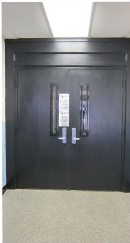
LEFT: Classrooms just past the office were equipped with locks from ASSA ABLOY Group brands: Corbin Russwin (door locks), Securitron (power supplies), HES (strikes) and Rockwood (latch guard). They automatically lock from the inside when closed. During an emergency, teachers have been instructed to keep their classroom doors closed until they hear a code phrase from a sheriff’s deputy. RIGHT: Security screens from Harmony Security Products were installed in front of the glass of several doors on campus. The stainless steel mesh screens are impervious to rips.
